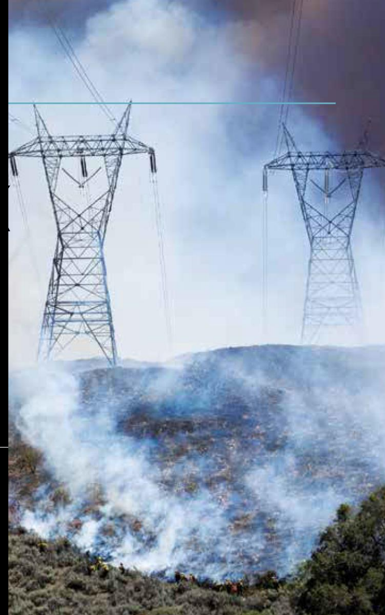
Source: Courtesy of the National Emergency Response - Autumn 2014
